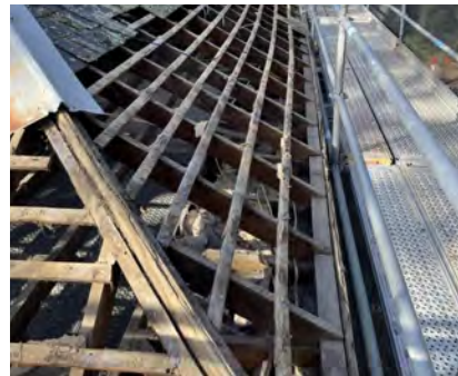
Roof structure exposed but not retained during deconstruction.
